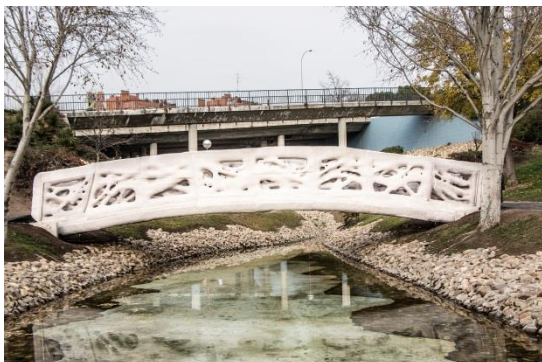
3D printet bro, Alcobendas, Madrid (Acciona/D-Shape tekn.)
