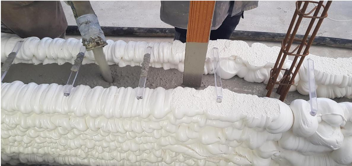
*Concrete pouring in between the polyurethane formwork.*
