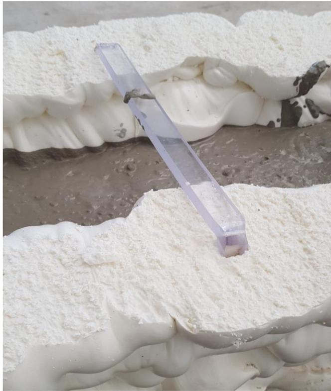
*Acrylic ties installed on top of the polyurethane foam.*
