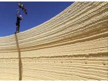
One of the latest projects of the Mediated Matter at Massachusetts Institute of Technology Media Lab is using a robot to 3d print large scale structures. The name of the machine is DCP – digital construction platform.
